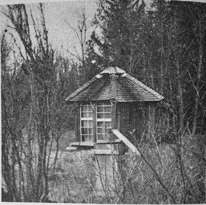
Hermit Matthew Casey built this round cell for himself. He got a bargain in two-by-four's, but they were all six feet long. So he used them as uprights in his dwelling, which is remote from the huts of other hermits.
