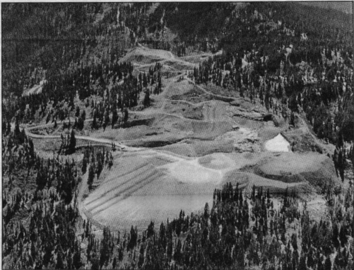
HERE'S AN AERIAL VIEW of the old mine site which the Tso lum River Restoration Society is only $4 million away from stopping leakage.
