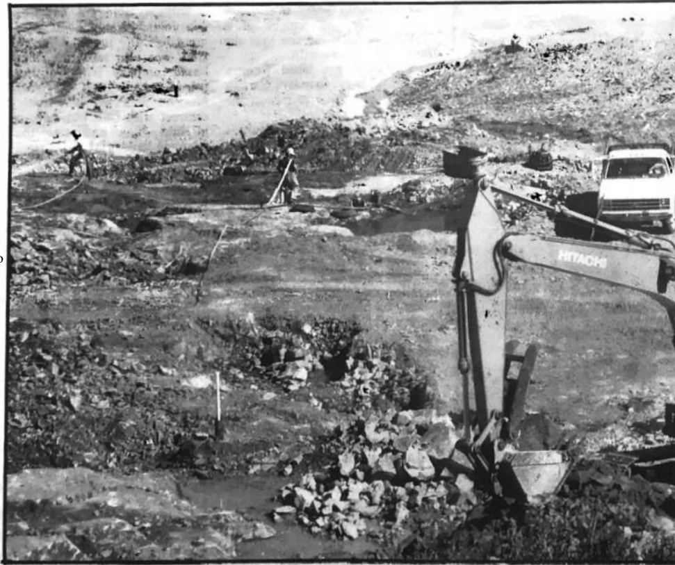
Crews at work 'washing' down pit floor of abandoned copper mine
