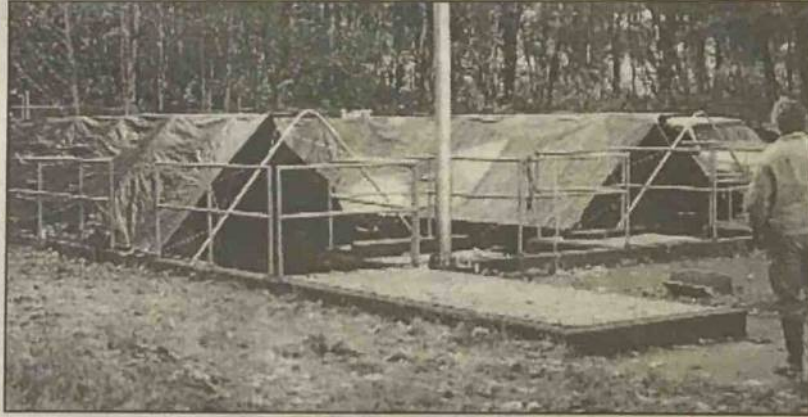
RACEWAYS, LARGE EIGHT-FOOT deep cement boxes, approximately 80 feet long, are covered to provide a dark place for fry so they don't crowd each other.
