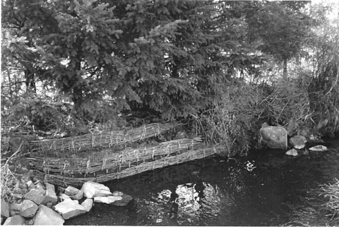
Figure B.1 Willow wattles constructed in Portuguese Creek July 1998.
