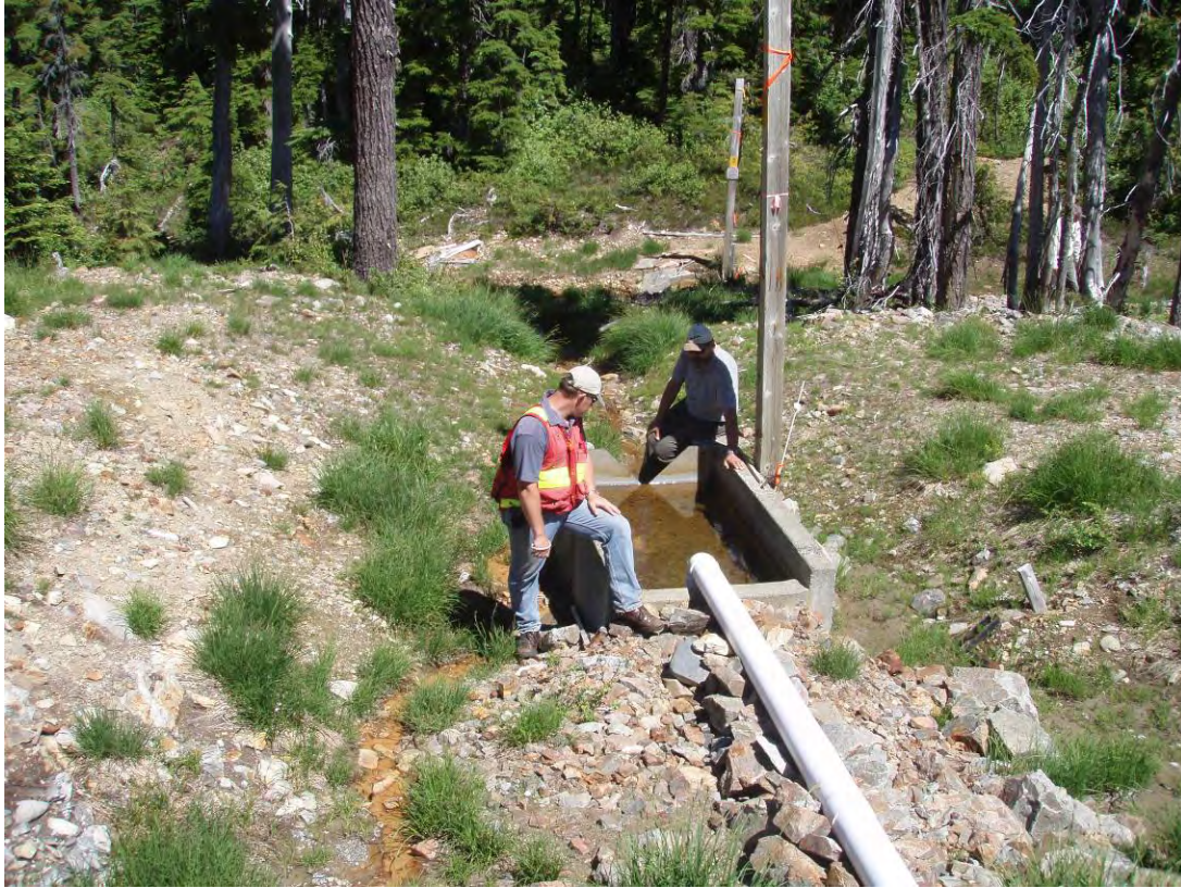
Photo 21: Weir 1 at toe of East Dump.
