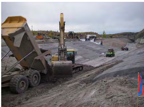
Baker Creek – Giant Mine Realignment Project – Liner Installation
