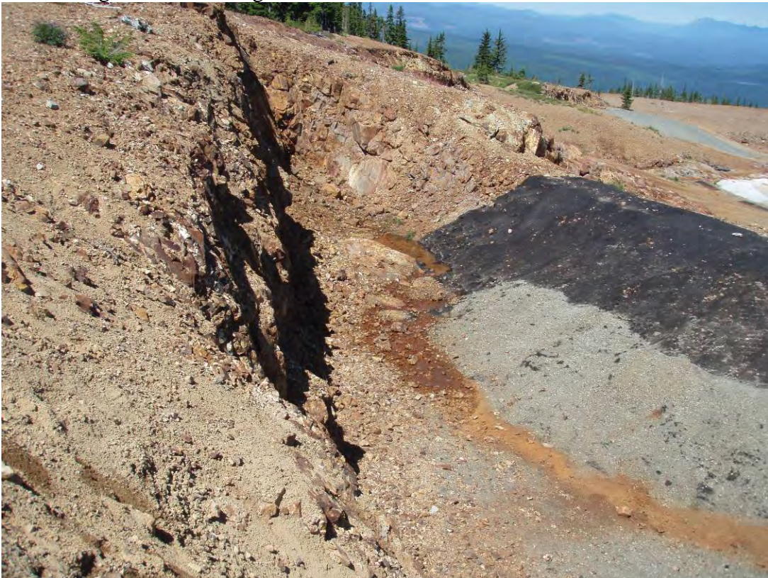
Photo 2: Pit wall at western perimeter of the pit adjacent to Seep 16.
