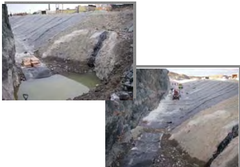
Baker Creek – Giant Mine Realignment Project – Liner Installation
