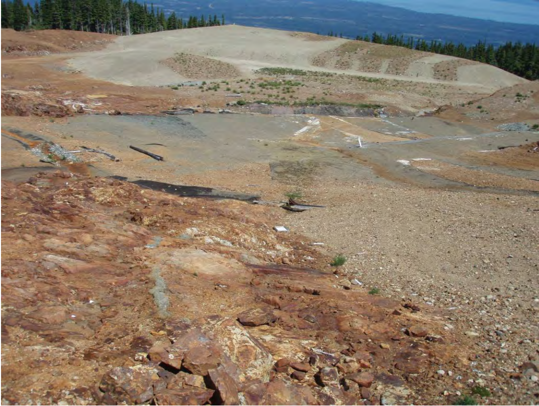
Photo 1: View east with covered East Dump background and asphalt impregnated geotextile in midground.
