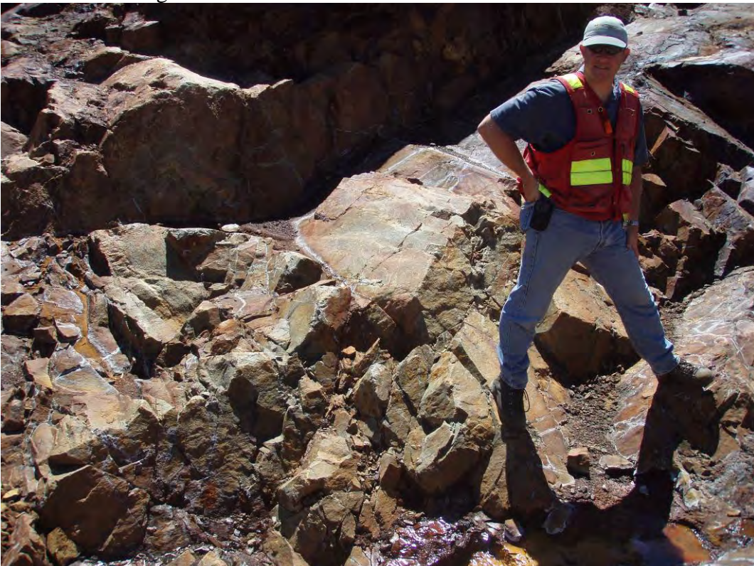
Photo 6: Irregular sharp and angular areas of the pit floor that will require significant site preparation.
