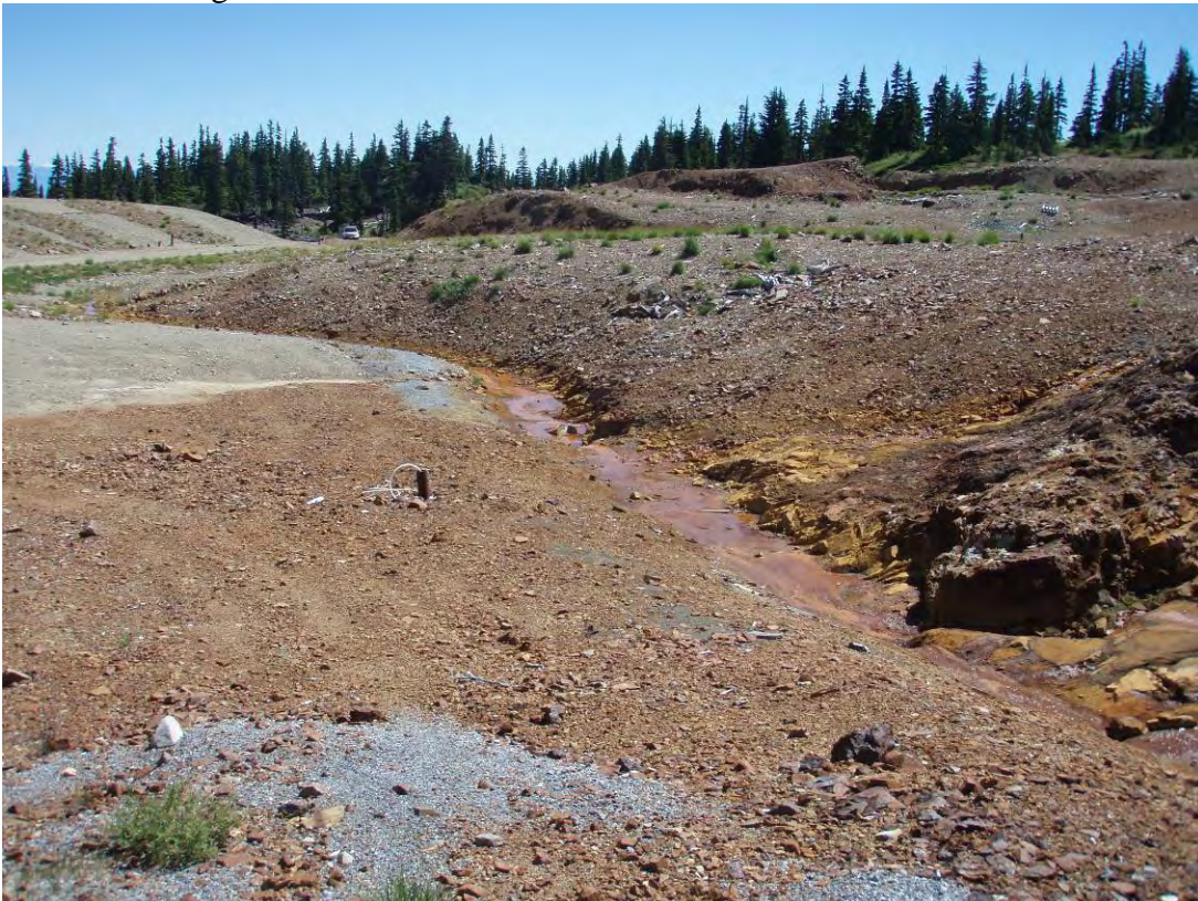
Photo 12: Upper seepage collection channel.
