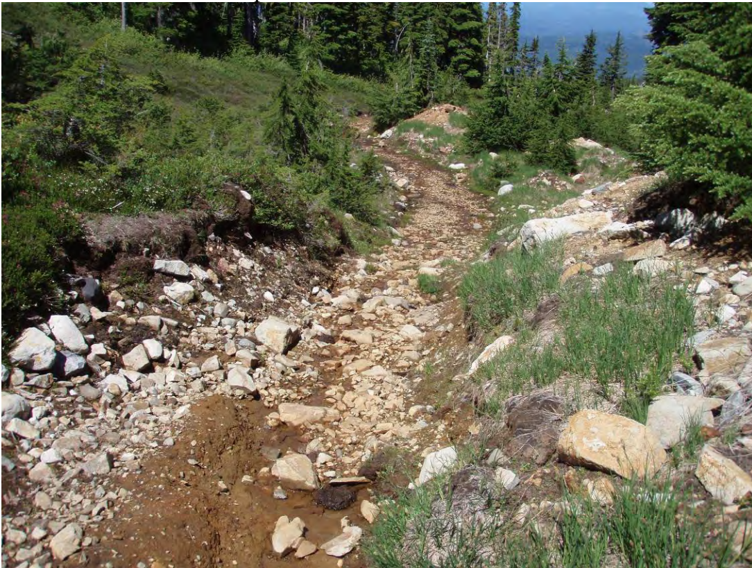
Photo 14: Uphill diversion ditch looking north.
