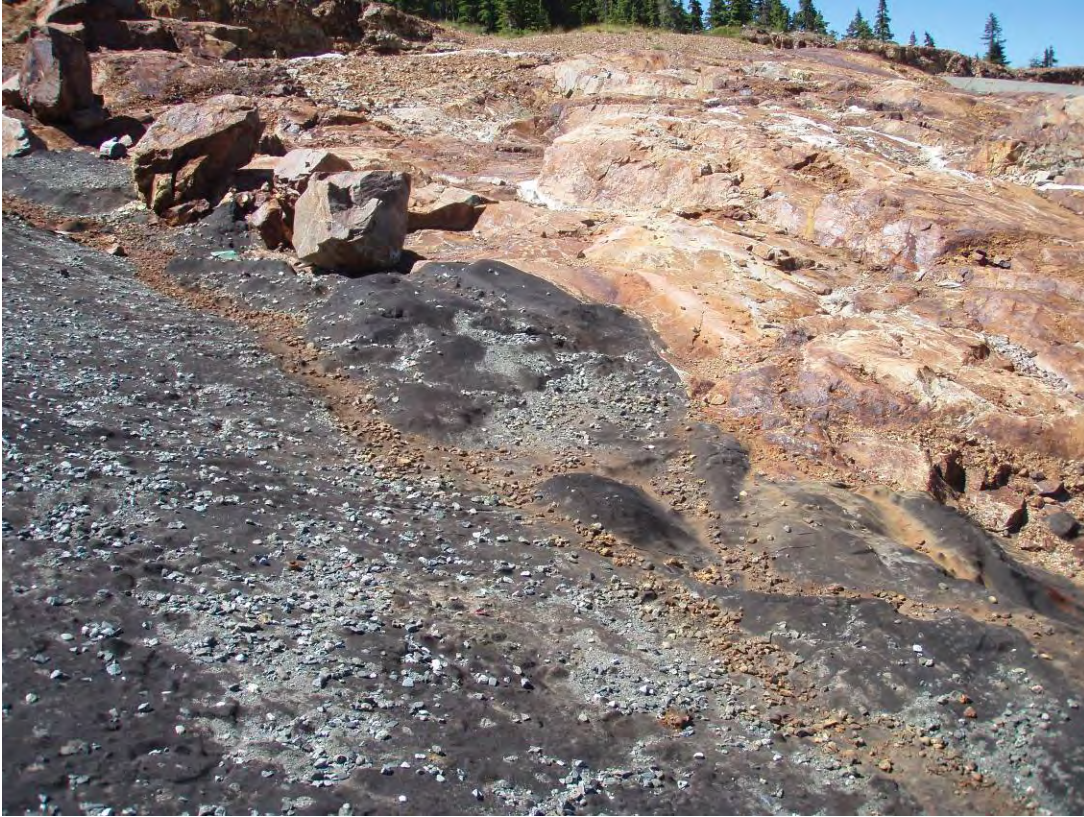
Photo 11: Washed areas of pit floor with bitumin impregnated geotextile in foreground.
