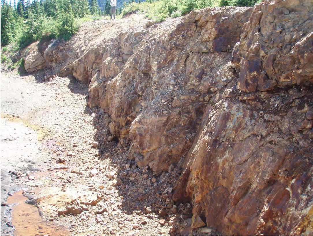
Photo 9: Pit wall requiring buttress fill prior to covering.
