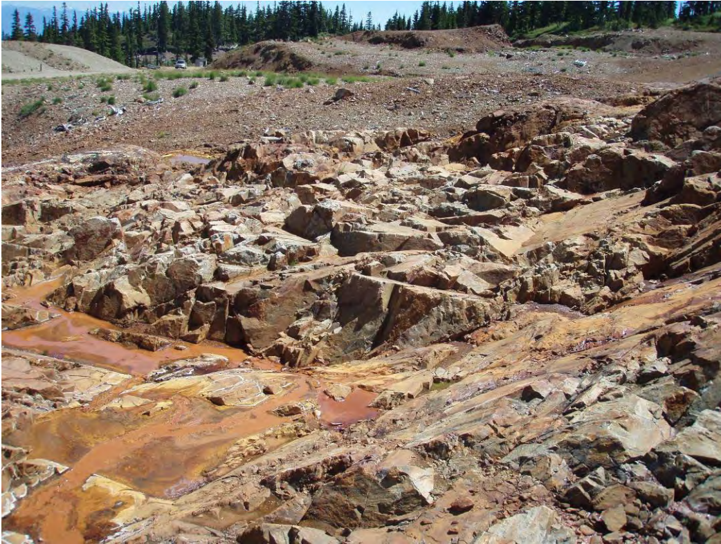
Photo 7: Irregular sharp and angular areas o the pit floor that will require significant site preparation.
