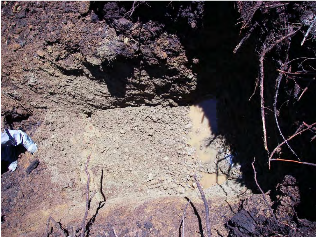
Photo 8: SRK-T-08-07 - Weathered Till with gravel; water seeping through.
