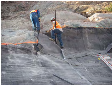
Baker Creek – Giant Mine Realignment Project – Liner Installation
