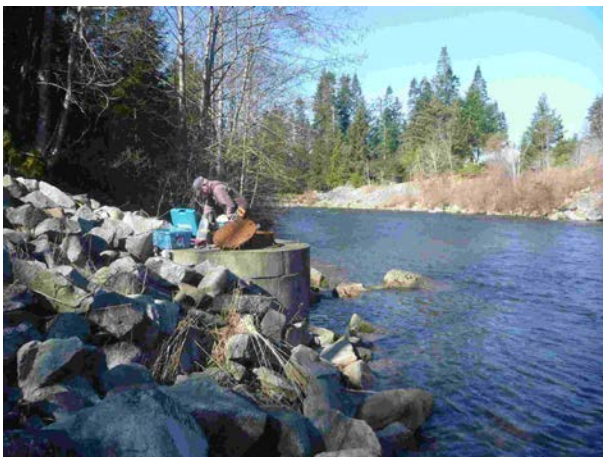
Photo 8. View upstream of the Oyster River mainstem showing the Sidechannel intake manhole where level logger "Intake" was installed. (April 1, 2014)
