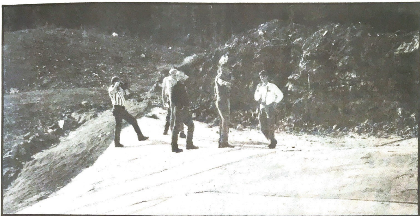
Field trip members view concrete cover poured on top of waste rock
