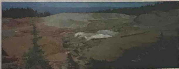
The former copper mine at the top of Mount Washington was capped once to prevent leaching. It will likely be capped again at a cost of approximately $5 million.
