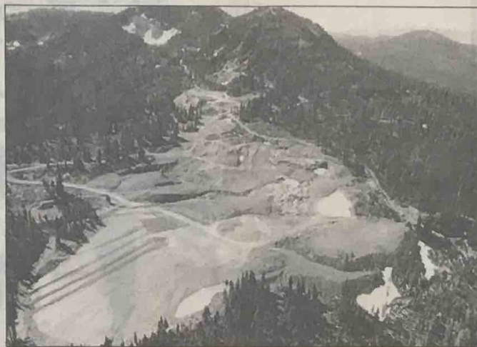
Mount Washington mine site: problems 30 years later
