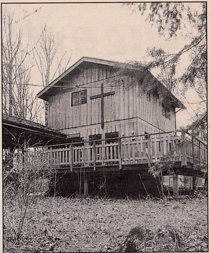
Brandt's 20' by 20' hermitage, now in Merville, is made of salvaged wood from old farm buildings. Photo by Boomer Jerritt
