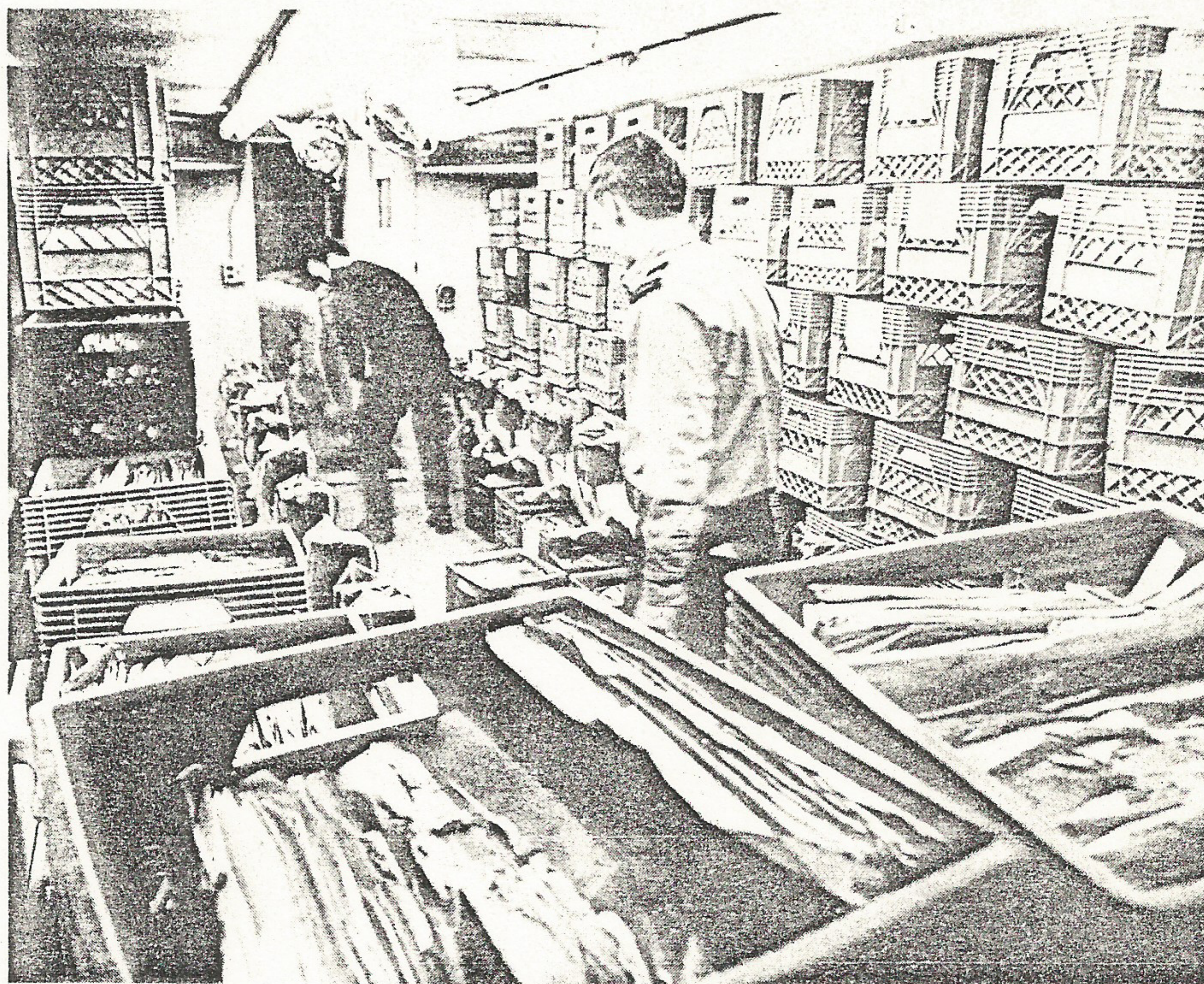
Crates of documents being placed in the chamber. Note the method of stacking the crates so as to allow maximum air circulation. ( The Winnipeg Free Press )
